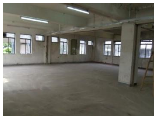
(1) Site formation works
