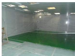
(5) Laying of a floor protection film
