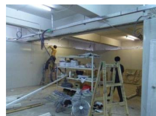
(4) Installation of indoor air-conditioning and lighting as well as major piping and wiring
