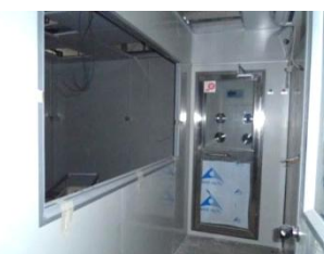
(3) Installation of an air shower room
