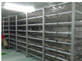
(6) Fixing of the frame and electric circuit for the cultivation racks
