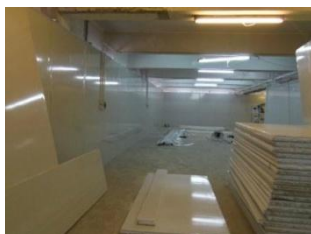
(2) Fitting of heat insulating panels
