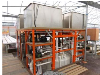
Specially-made storage, cooling, delivery and filtering devices for the nutrient solution
