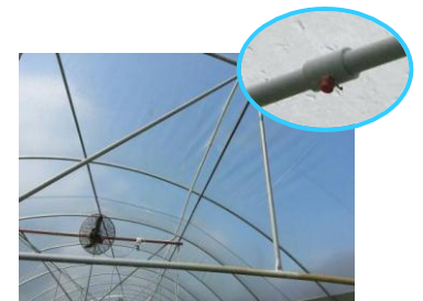
Using fans and misting equipment to cool the greenhouse in summer
