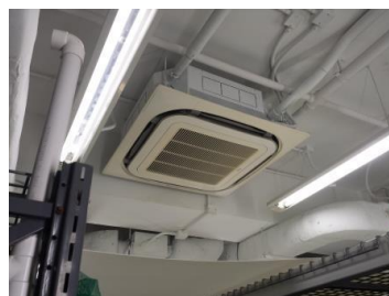
Temperature controlled by room air-conditioners
