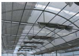
Shading nets and mist sprayers
