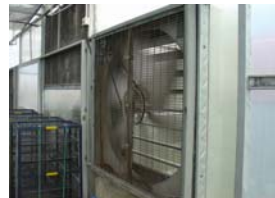
Powerful ventilation fans
