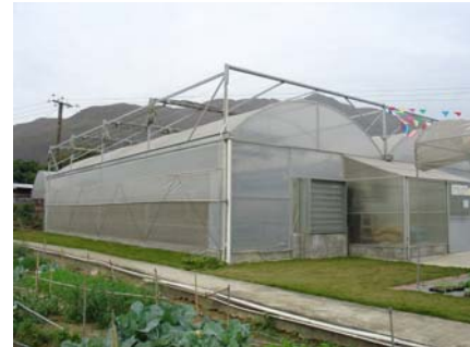
External view of completed greenhouse
