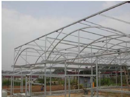
Construction of greenhouse in progress
