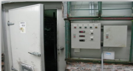
Display panels outside the mushroom cultivation room showing different indices and the operation of facilities
