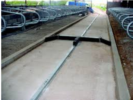
27. Automatic Scraper System For removal of livestock waste automatically.
