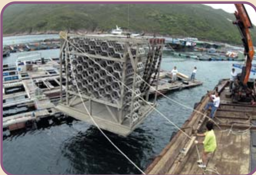
附有青口的人工魚礁安放在魚排 旁的水域 An artificial reef with shellfish being unloaded beside a fish raft
