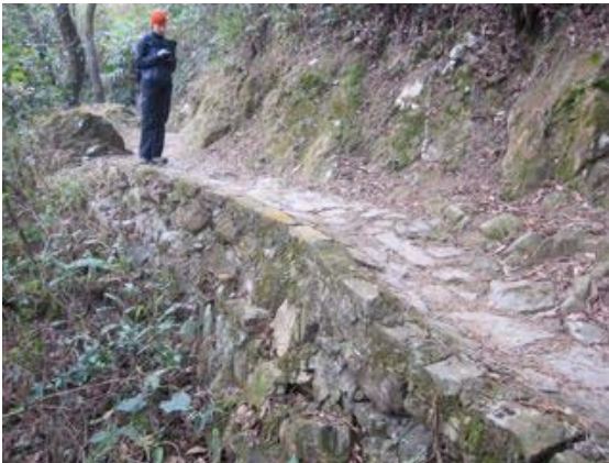
Sustainable sections of the Ho Pui Trail: existing rock wall and tread armoring (left) and nice section of benched tread with natural rock edges that define the trail (right).
