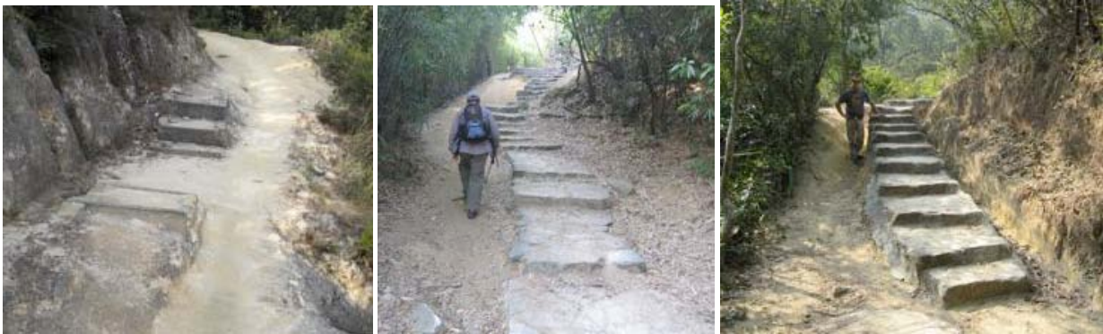
Steps placed for erosion control are ineffective and creating trip hazard; users have simply widened the tread to go around them. Erosion continues, user experience is degraded, and safety becomes a concern.
