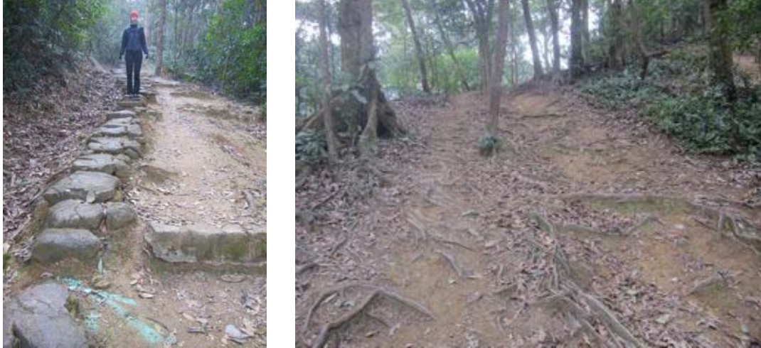
Start of the Ho Pui Trail: steep, fall-line section with severe erosion (left) and numerous social trails (right). This section needs to be rerouted and closed.
