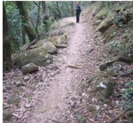
Sustainable sections of the Ho Pui Trail: existing rock wall and tread armoring (left) and nice section of benched tread with natural rock edges that define the trail (right).
