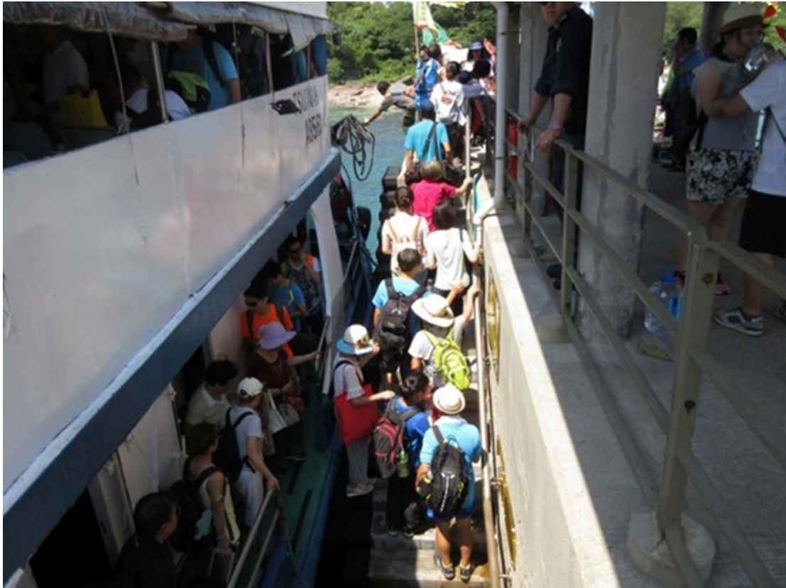
Figure 3.5 Existing Narrow and Steep Landing Steps of Tung Ping Chau Public Pier
