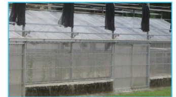
A greenhouse with polycarbonate sheets replaced
