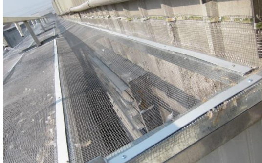
26. Water Spraying system For avoiding feather blowing out from rearing sheds by the exhaust fans.
