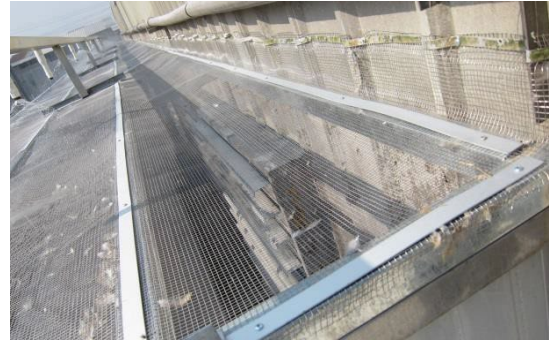
26. Water Spraying system For avoiding feather blowing out from rearing sheds by the exhaust fans.
