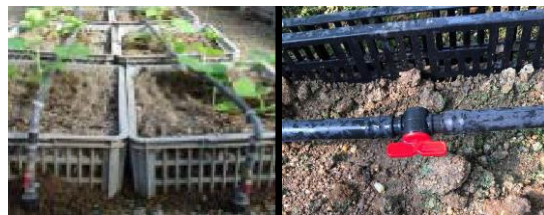
18. Parts and materials for irrigation system For setting up irrigation system.
