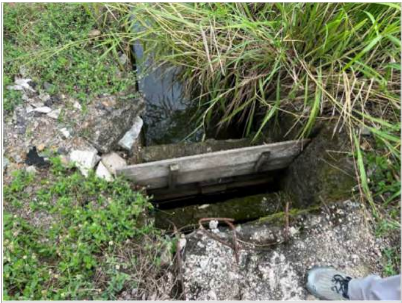
Concrete Gate with Wooden Board
