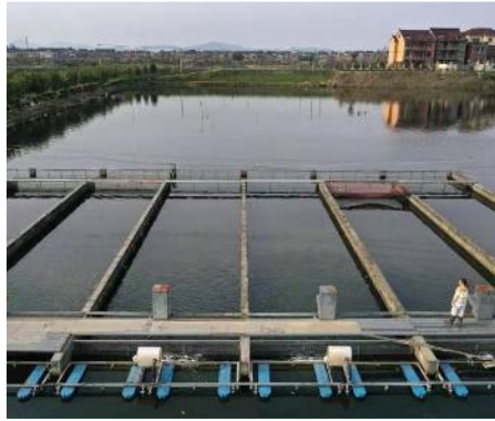
In-pond raceway system
