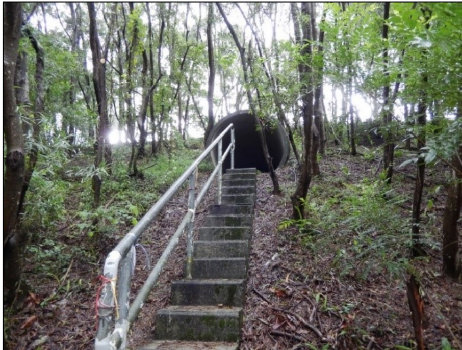
Figure 7. The first wildlife underpass in Hong Kong beneath Route 3 was constructed in 1998.
