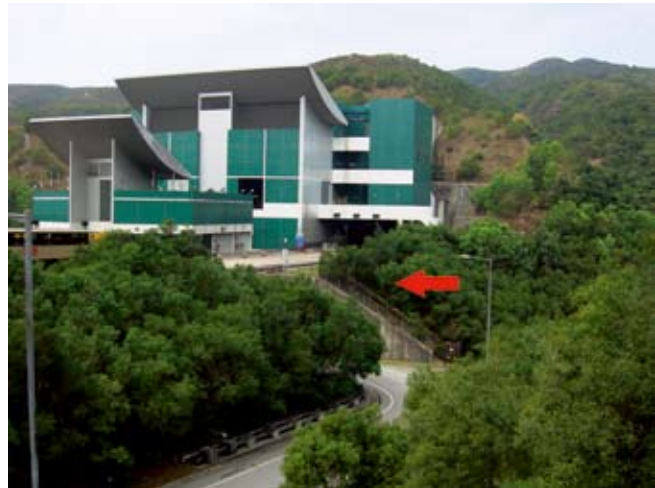
Fig 15. Location of the entrance (red arrow) of the animal crossing.
