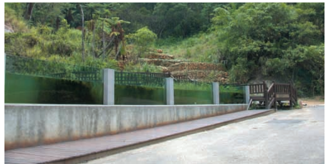
Figure 6 Concrete and reinforced glass wall of the artificial wetland.
